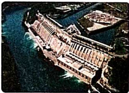
Hydroelectricity power plant
